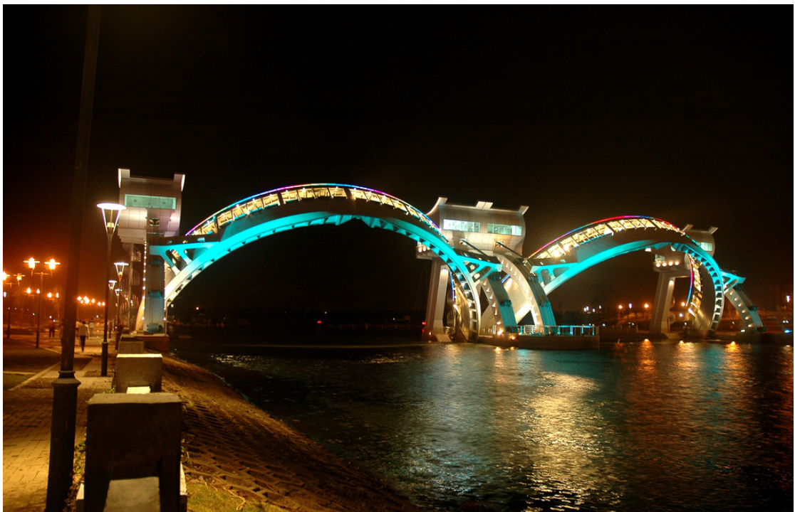
Pic. 2 The Sanchahe River Sluice
