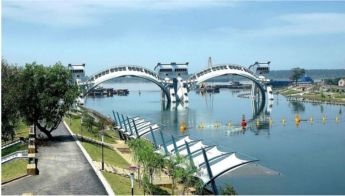
Pic. 1 The Sanchahe River Sluice
